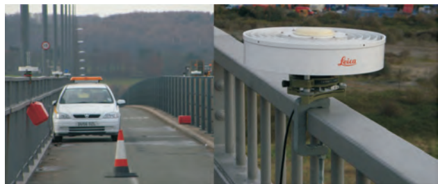
Fig. 28. Four of the five survey points on the Bridge (left), and a close-up of location C (right), all using Leica lightweight At503 choke ring antennas on the Avonmouth Viaduct.
